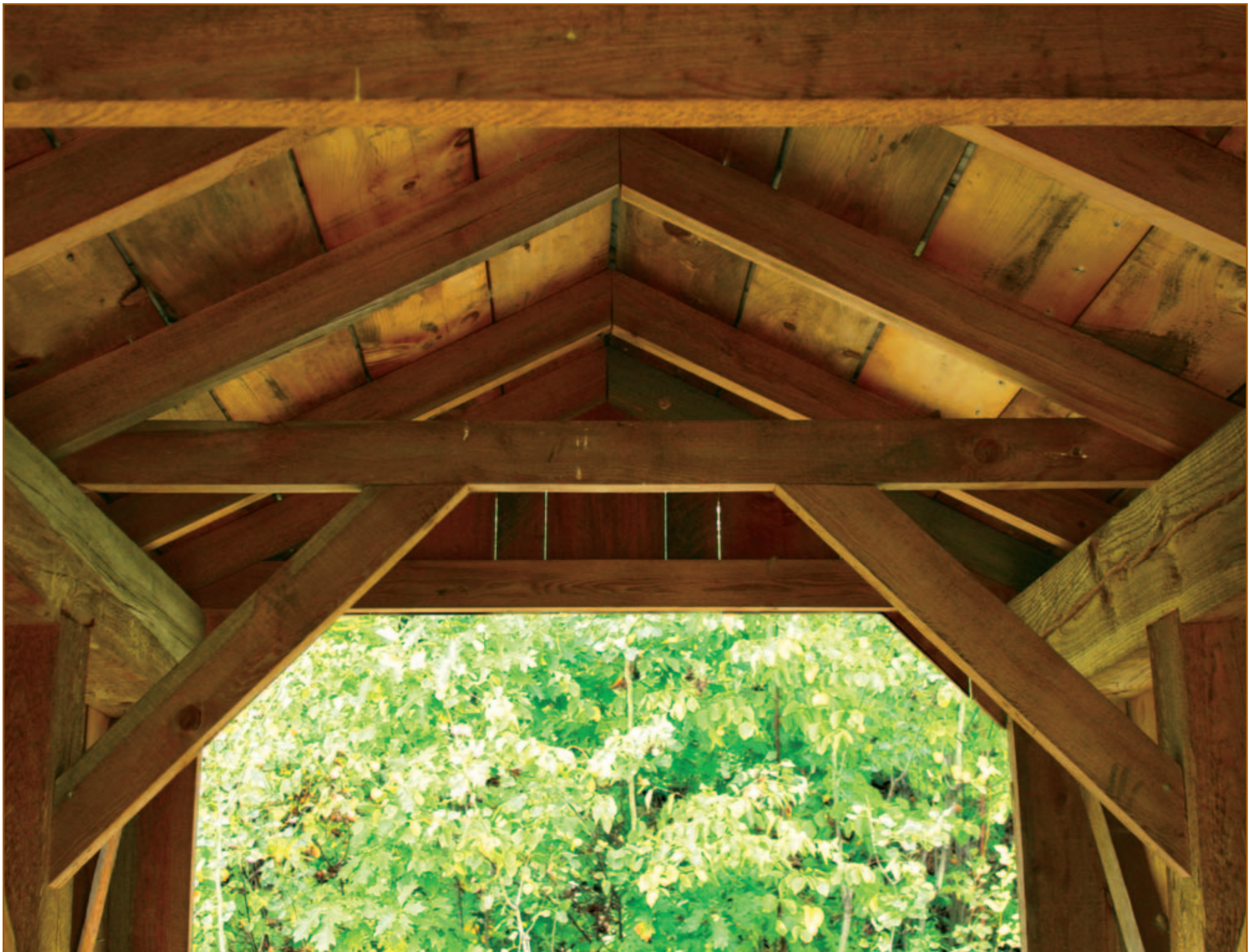
Old wooden covered bridge: Bala cranberry farm
